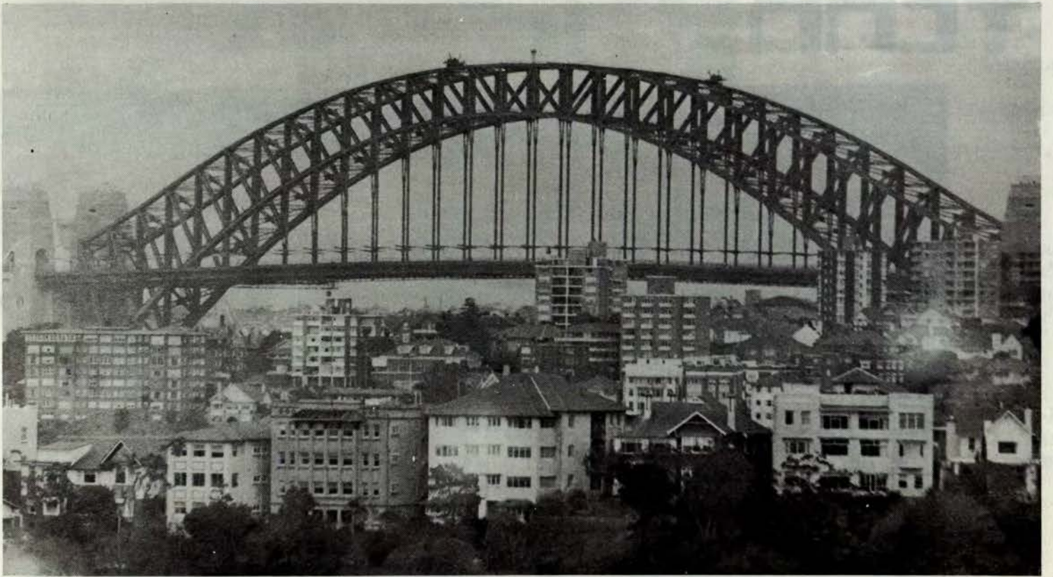
That's a strange place to build a bridge (by G. Maddock)
