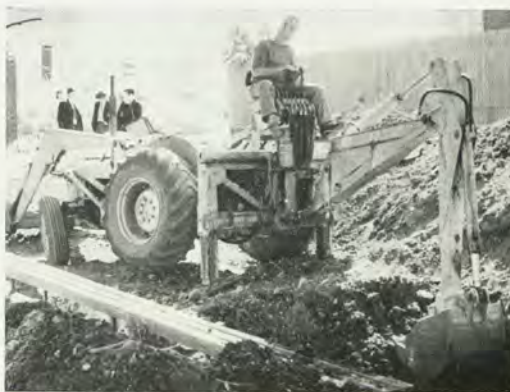
BACK-FILLING FOR THE NEW CAR PARK
