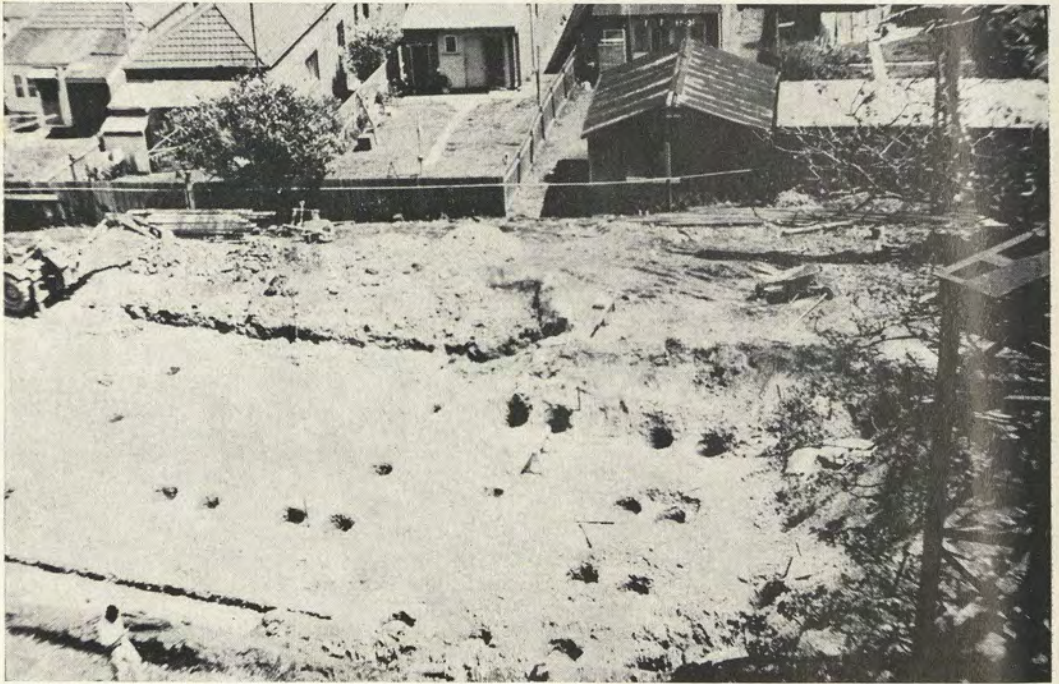
Holes are drilled for foundations.
