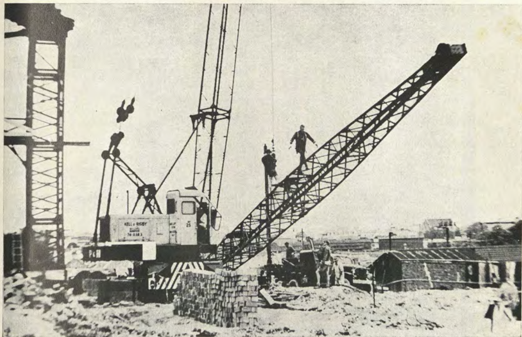
The all-important crane is assembled.
