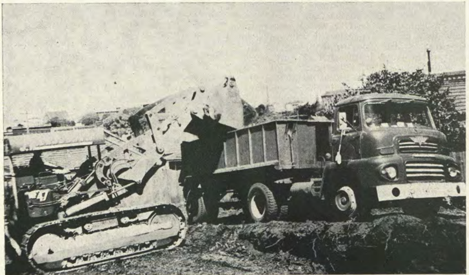
Heavy machinery clears the site.
