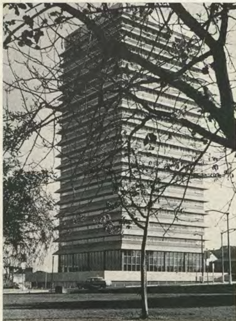
I.B.M. BUILDING, SYDNEY
