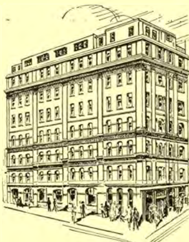
M.B.C. Building, 6 Dalley St.
