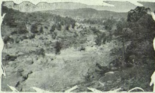
SITE OF WYANGALA DAM, NOW UNDER CONSTRUCTION
