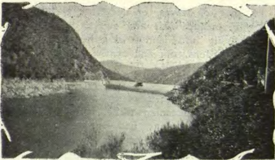
WALL OF BURRENJUCK DAM, LOOKING DOWN RIVER.
