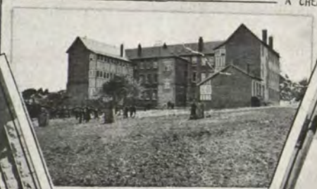
SCHOOL - REAR VIEW.
