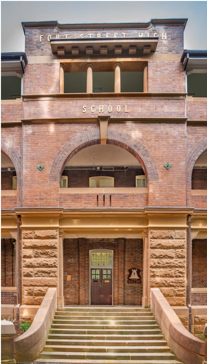
Completed front façades of Building A including stone and brickwork.
